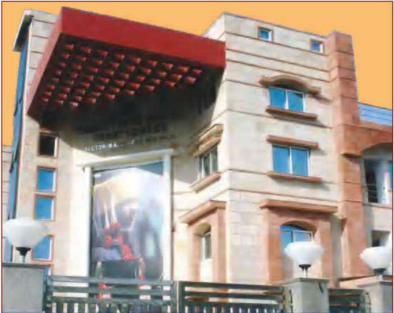
Tribal Youth Hostel, Chhattisgarh Sector 18A, Dwarka, New Delhi
